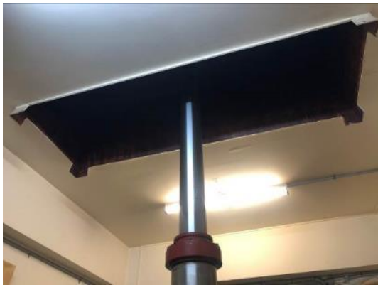
Figure 384: Detail view of hydraulic coffin lift from lower ground floor to altar level.
