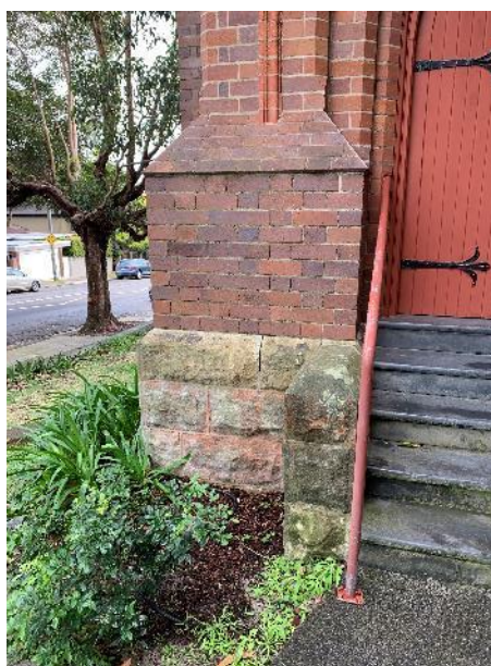
Figure 194: View of stone footings to church
